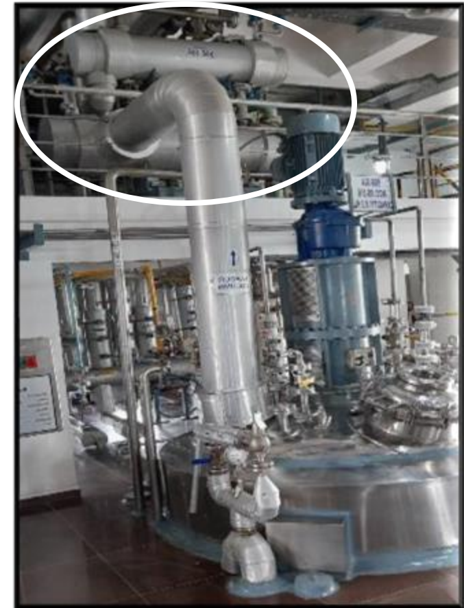
Reactor vent connected with double condenser
