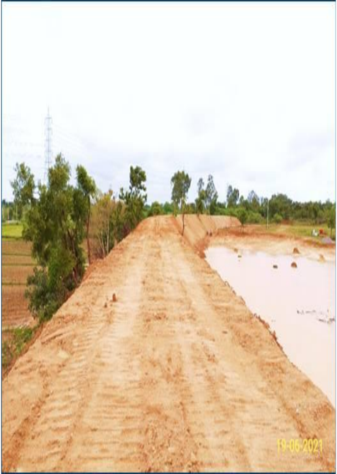
Bund Strengthening after
