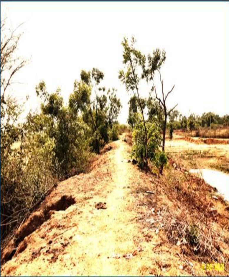
Bund Strengthening before
