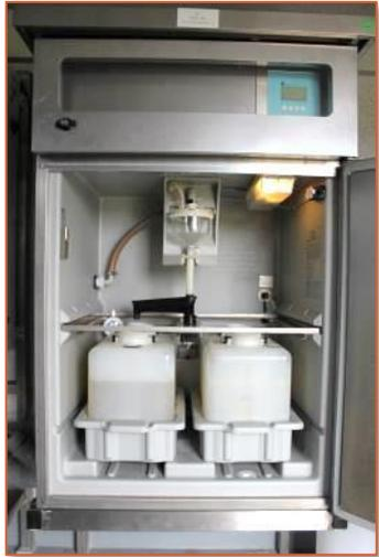
Automatic sampling device for composite samples
