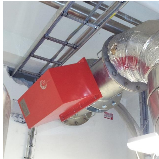
Active flap valve 蝶阀
