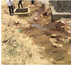
Groundwater collection and runoff
