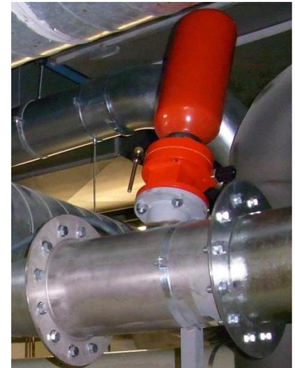
This is normally combined with a fast acting mechanical valve or a chemical barrier to protect the dirty side pipes
