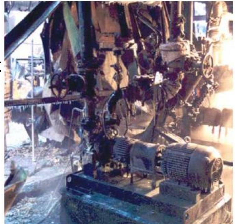
Incident: explosion of pumps as a result of overheating
