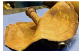
Tank bottom after explosion shows weld seam and thinned original bottom head.
