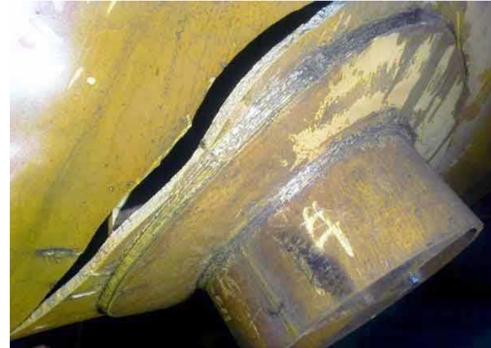
Image of bottom of pressure vessel
