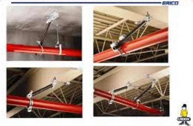
Fire Sprinkler Earthquake Protection – Sway Bracing
