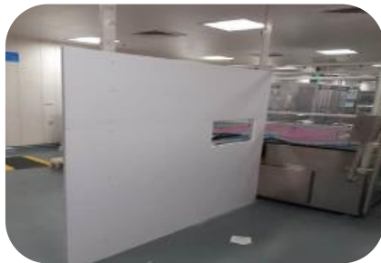
Partitions in inspection areas
