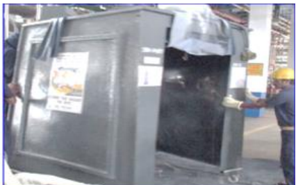
8. Arranging the Enclosure.
