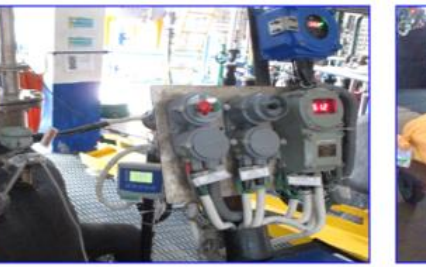
10. Ensuring the earthing continuity on online earth monitoring unit.
