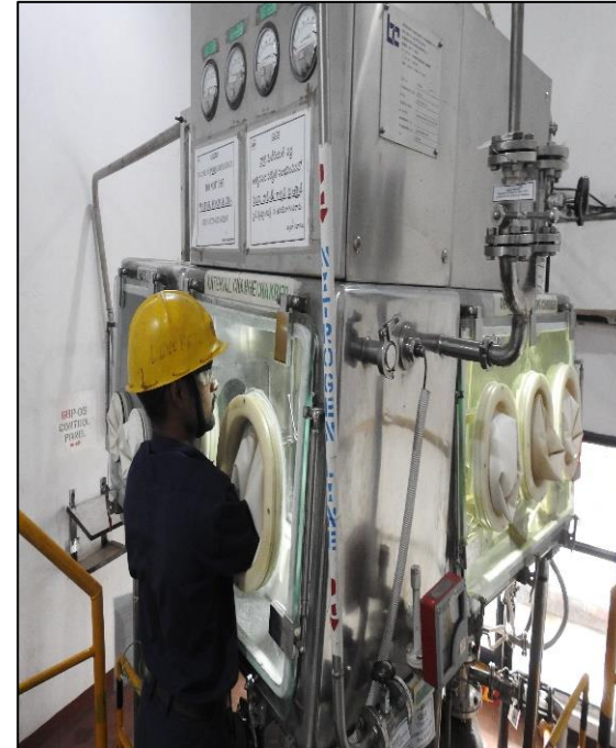
Charging through Isolator
